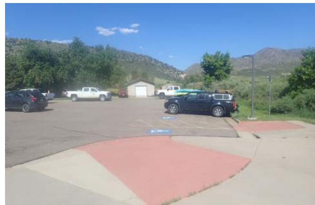
VISITOR CENTER TRAILHEAD ACCESSIBLE PARKING
