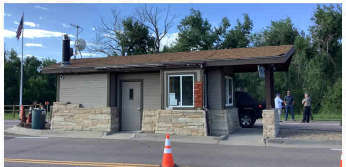
Existing Entry Gatehouse
