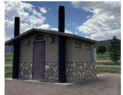
Example Image of Vault Toilet
