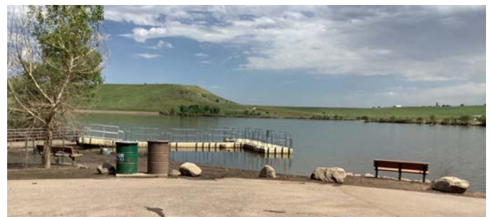
Bear Creek Reservoir Existing Boat Ramp
