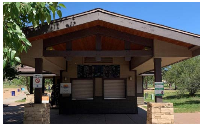
Existing Condition of Food Concessions Exterior
