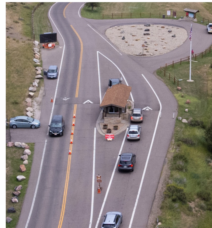
EXISTING ENTRY GATEHOUSE
