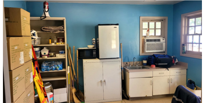
Existing Condition of Ranger Station Interior
