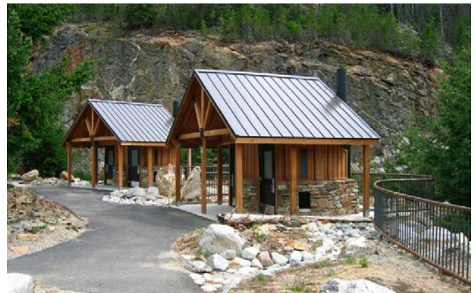
Example Image of Vault Toilet
