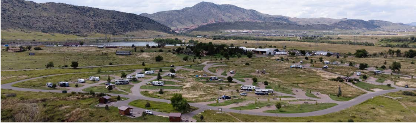
Overall View of Existing Campground
