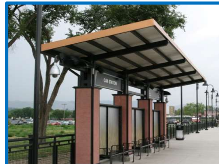
Improvements to RTD Shelters
