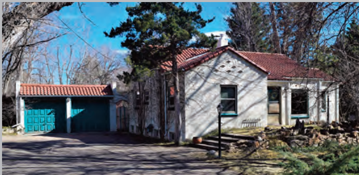
Similar to Spanish Colonial style, but plainer and more modest. Tile roof is distinguishing feature. Common elements: heavy tile roof, low pitched gable or hipped roof, wrought iron grille work, arcaded entrance/porch, stucco finish, casement window, arched entrance/window. (Image: 1090 Pikeview St.)
