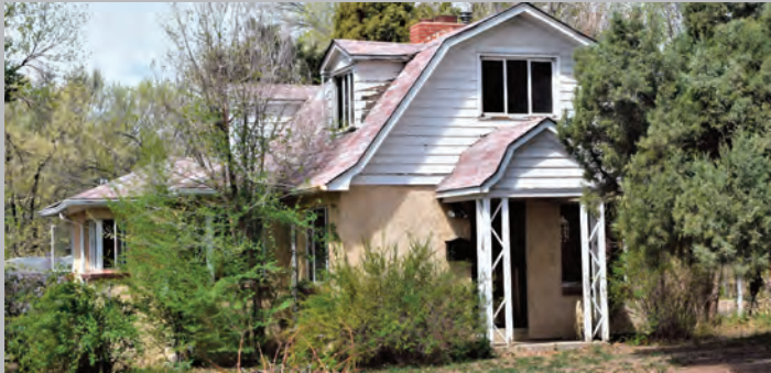
Barn-like gambrel roof is distinguishing feature of this sub-style of Colonial Revival. Common elements: gambrel roof, wide overhangs, gable end chimneys, round windows in gable end, steep stepped gable, porch under overhanging eaves, 8-over-8 windows, dormers (Image: 1215 Wadsworth Blvd.)
