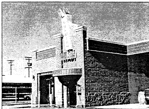
Encourage design of new commercial buildings that reflect the early auto influences on West Colfax.
