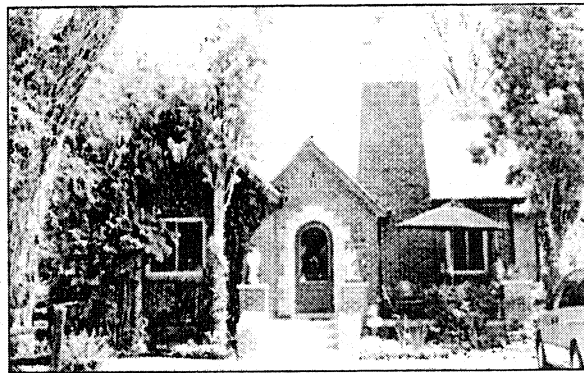
There are several excellent examples of the English Norman Cottage, shown at right 1560 Ames Street, 5JF3584. Photo by Cathleen Norman, 2003
