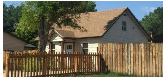
Side gabled (roof) house
