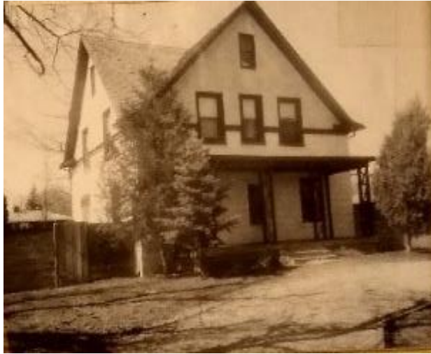
5JF.7666/1821 Dover Street, photo taken in 1969. This 1908 farmhouse was included in this survey. The early residence is associated with the Jellison Family.
