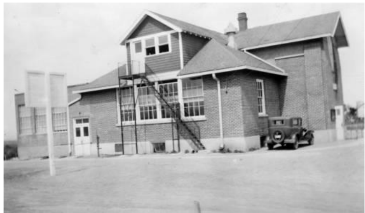
5JF.7698/6001 W Mississippi Avenue, the former Bancroft school, as it was in 1940. Although now a commercial building, the former school is the only education-related resource included in this survey. Image: Denver Public Library.
