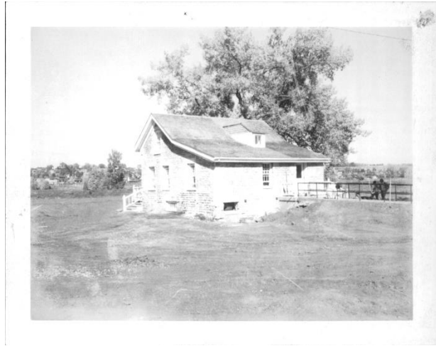
Photo of the Stone House taken immediately following its renovation in 1976. The Stone House is the oldest extant house in Lakewood. Image: Heritage Lakewood Belmar Park, City of Lakewood.
