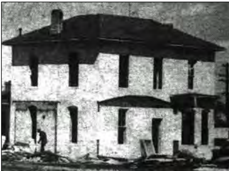
Figure 6. Civil War veteran John Robb constructed this large house (no longer extant) at the northeast corner of Carr Street and West Colfax Avenue in 1876. SOURCE: Autabee and Autabee, West Colfax Survey , 49.
