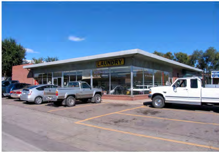
5JF.6527 – Looking Northwest at southern facade. Scotch Wash Laundry. 1565 Carr Street. Photo ID: 5JF6527a. September 2014.
