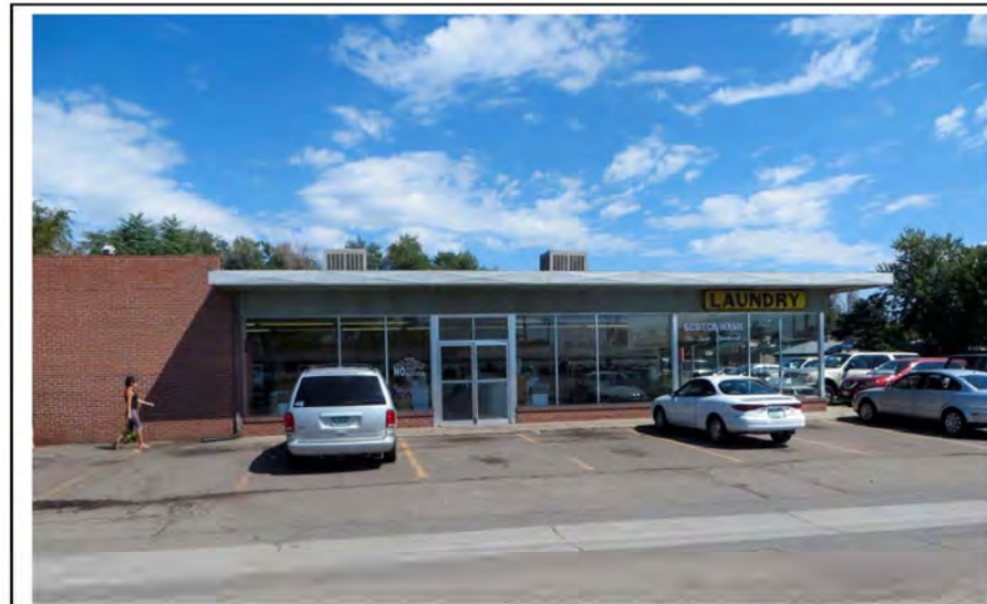
5JF.6527 – Looking North – Southern Facade. Scotch Wash Laundry. 1565 Carr Street. Photo ID: 5JF6527d. September 2014.
