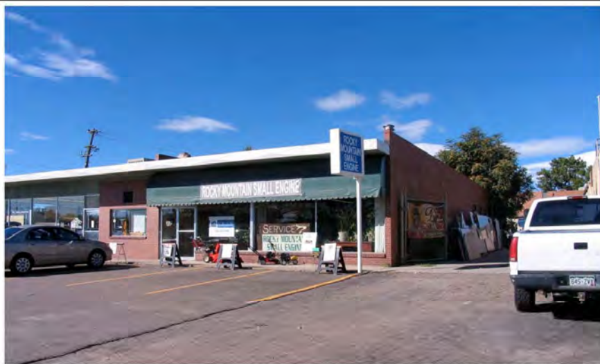
5JF.6527 – Looking southwest at eastern facade. Scotch Wash Laundry/Rocky Mountain Small Engine. 1565 (1575) Carr Street. Photo ID: 5JF6527b. September 2014.
