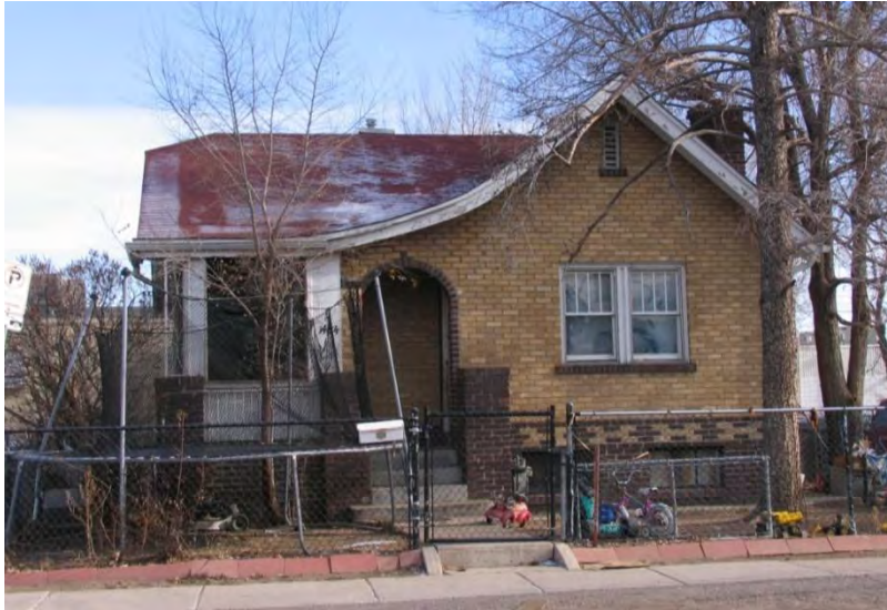
By the 1920s, Lakewood's Mountair neighborhood began to see houses constructed in materials beyond horizontal wood siding. This English Norman style home at 1484 Ames is one of the residences that broke away from the popular Craftsman style from a previous generation. (Photo: Robert Autobee).
