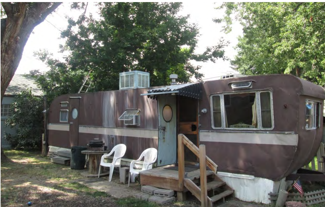
The corridor for the West Colfax Avenue Historic Resources Survey includes two trailer parks. Both parks contain trailers and other contributing features more than 50 years old. (Photos: Robert Autobee).
