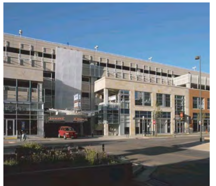
Parking access via side and rear streets
