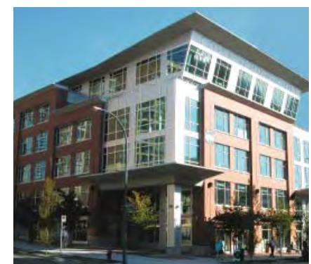
Building corner treatment
