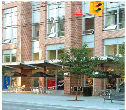
Shading structures for pedestrians
