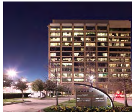
Well integrated entry and parking design; Tenet Health, TX
