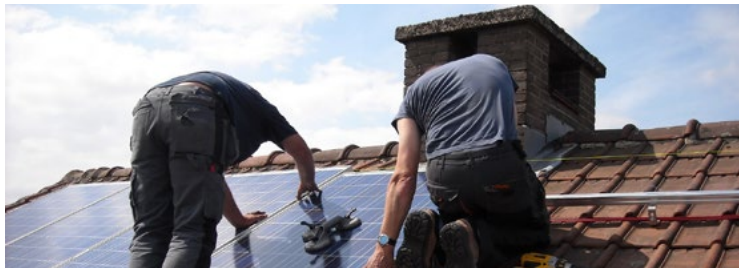
Requirements for a solar ready zone to preserve space and reduce the cost of future solar installation
