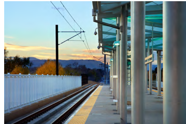
Lakewood Light Rail Station
