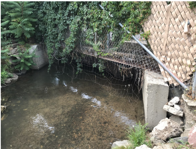
Existing culvert crossing
