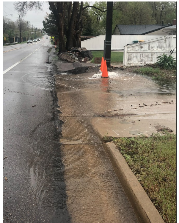
Existing flooding on 20th Ave.
